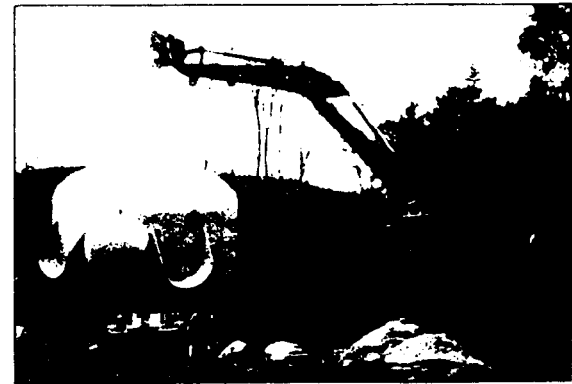
An ES10 shelter about to be lowered into the ground.
